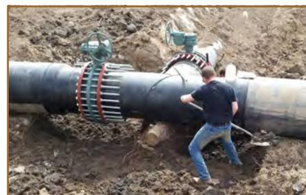
As part of RCPP project, the Lindell Diversion and Ditch Removal Project is 90% completed. 9,200 feet of buried PVC pipe was installed. This replaces above ground mainline and two pivots replaced a combination of hand line and big gun application systems.
